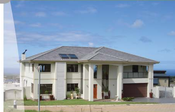
Retrofit of Existing Geysers ↑
